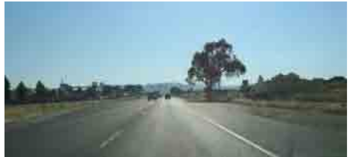
View of westbound SR 46 approaching Golden Hill Road
